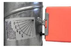
The minimum position screw can also be used to determine the damper position. The setscrew is aligned with the position of the damper blades. When the setscrew is in line with the duct, pointed at the Closed on the minimum position label, the damper is actually open. When it is hidden behind the motor and stopped against the anti-rotation post on the motor, it is Closed or at the minimum position.
